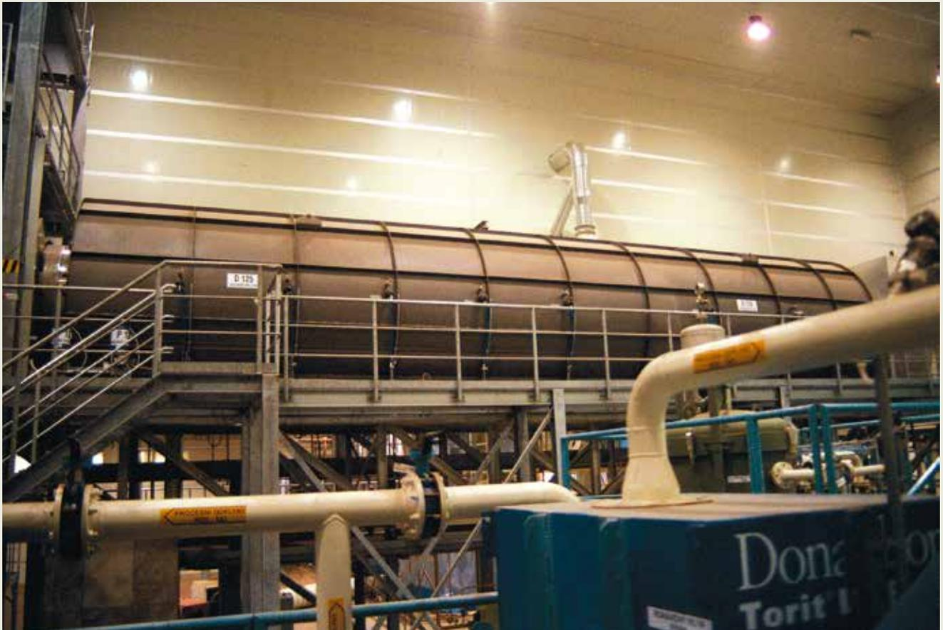
*Indirect thermal desorption unit in Spolana Neratovice served for evaporation of persistent pollutants from contaminated debris and soil into processing oil.*
