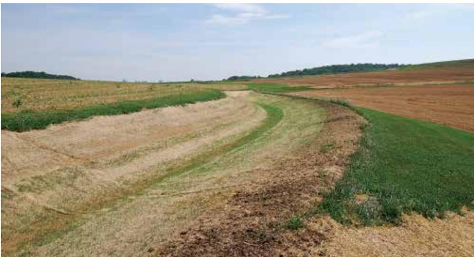
Counter erosion ditch
